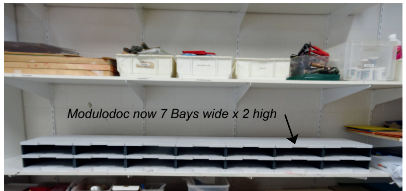
Installation at Rainworth SS
